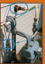
Example of a correct bond location for the gas house piping
