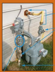
Do Not Bond to BGE Metering Equipment (electrically isolated) Gas House Piping (bond to this piping)
